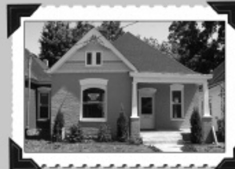
416 Johnson Avenue – After
