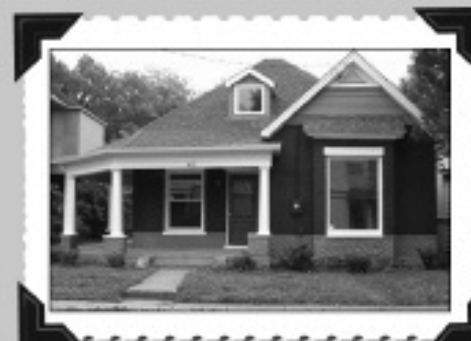
422 Johnson Avenue – After
